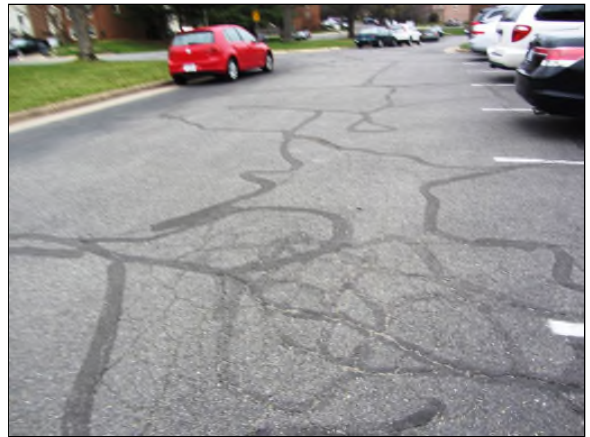
Photo #52. Alligatoring asphalt pavement.
