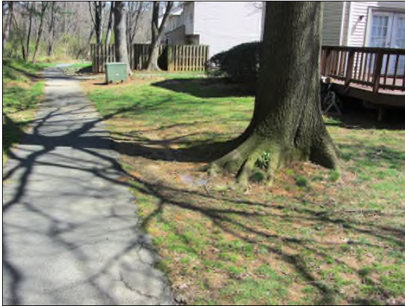
Photo #67. Tree roots are damaging the asphalt trail.
