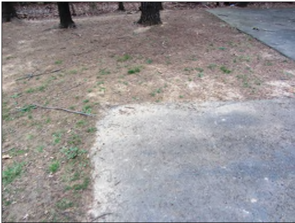
Photo #21. Defective grading adjacent to multipurpose court.
