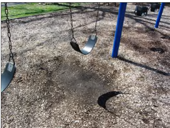
Photo #59. Inadequate resilient surfacing in the east tot lot.
