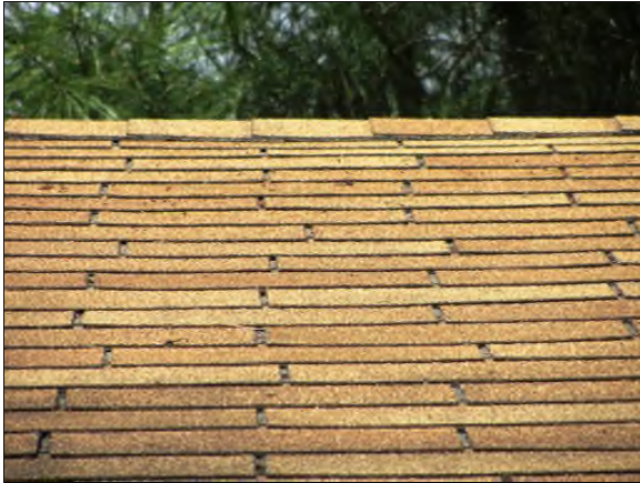
Photo #79. Asphalt shingles on shelter near the tennis courts are not properly aligned/installed.
