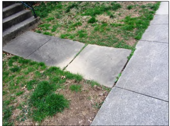
Photo #10. Defective lead walks are assumed to be unit owner responsibility.
