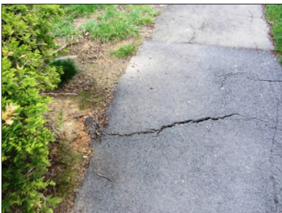
Photo #35. Typical damaged asphalt trail.
