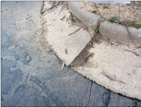
Photo #33. Typical displaced concrete curb & gutter.
