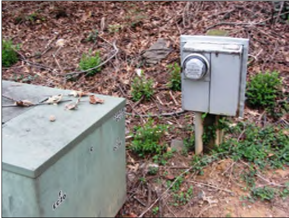
Photo #7. Electrical service is mounted too close to the ground.
