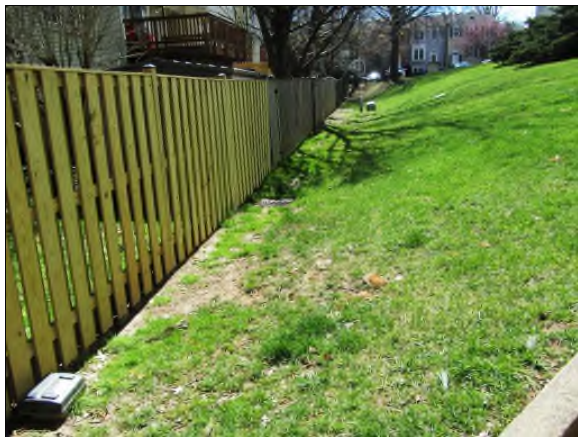
Photo #75. Typical open space behind units that has not been properly graded to move water to the stormwater system.
