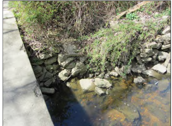
Photo #56. Damaged edge of concrete are likely a where safety railings were once attached.
