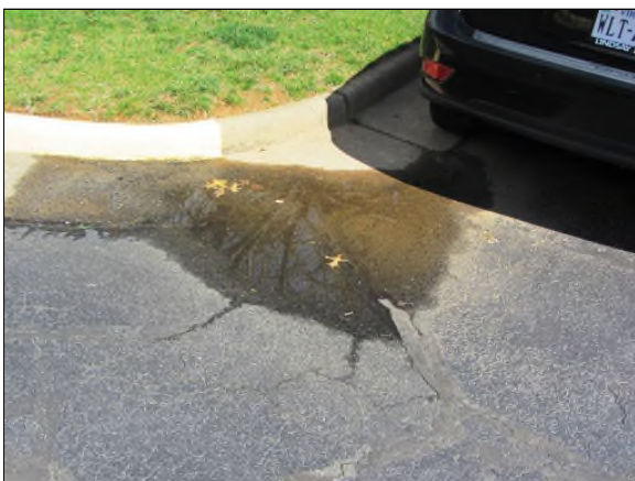
Photo #65. Depressed asphalt pavement and concrete curb & gutter impounds water and likely indicates damage to base materials and bearing soils below.
