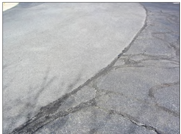
Photo #66. Alligatored asphalt pavement adjacent to a patch will result in the patch having a reduced economic life.
