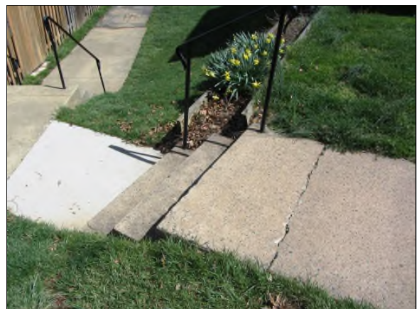
Photo #60. Handrails installed along exterior concrete stairs. Note crack immediately above the stair.
