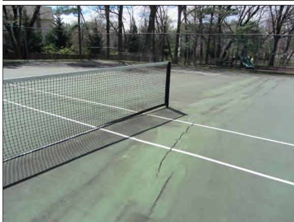
Photo #77. Patching of failed tennis court base asphalt is expensive and ineffective at extending the life of the court.
