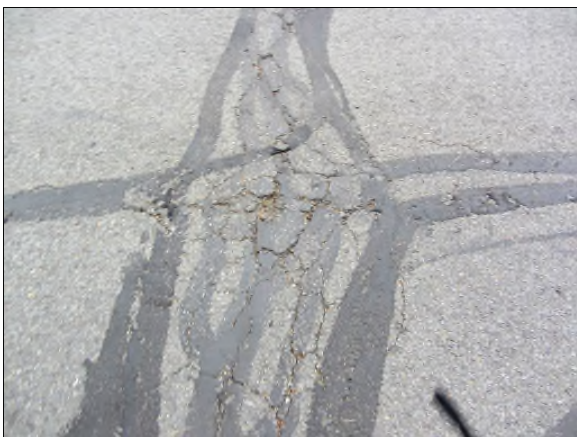
Photo #29. Typical cracked and alligatored asphalt pavement with ineffective crack sealing.
