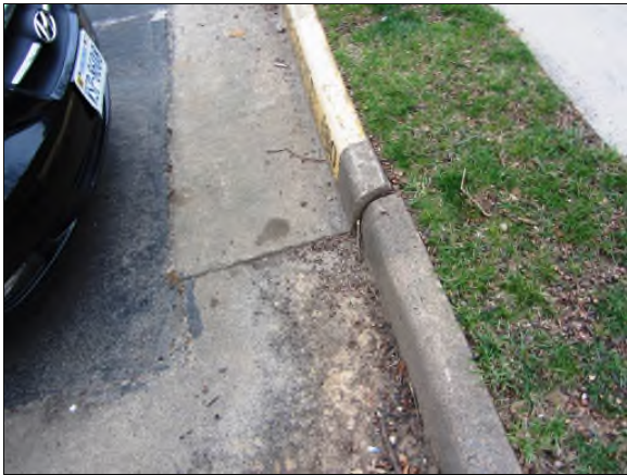
Photo #27. Typical displaced concrete curb & gutter.
