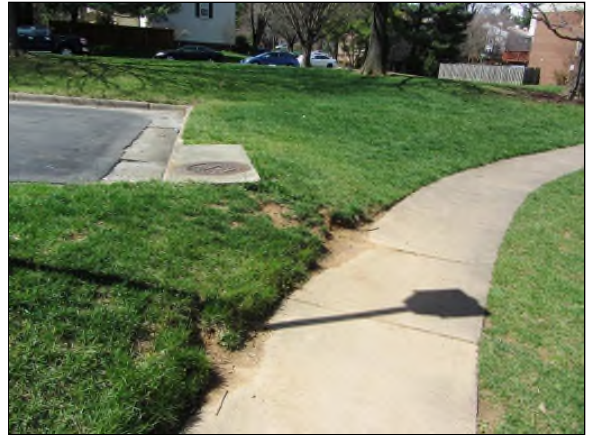
Photo #62. Defective grading adjacent to concrete sidewalk.
