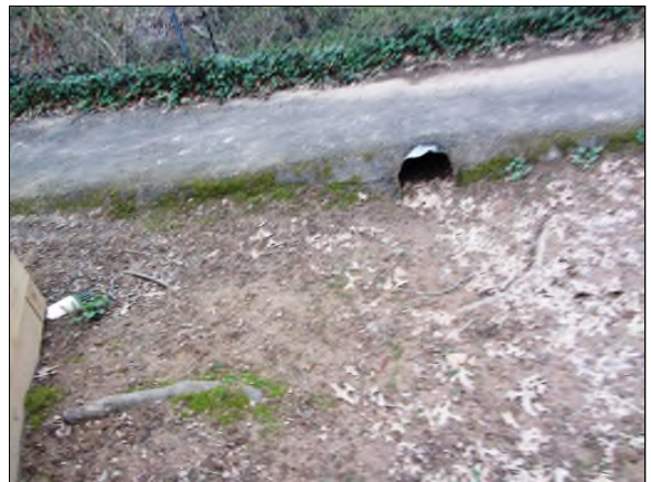
Photo #24. Lack of ground cover and inadequate pavement thickness above culvert.
