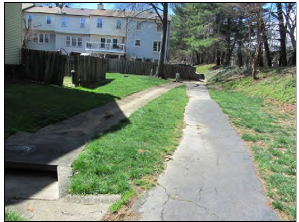
Photo #70. Concrete drainage swale adjacent to the asphalt trail, but the asphalt trail is still collecting water.
