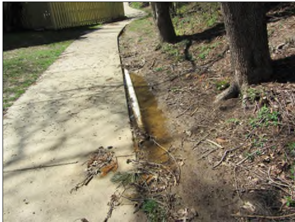
Photo #73. Defective grading (and apparent drainage project) adjacent to concrete pavement.
