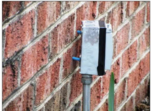
Photo #2. Electrical outlet at entrance feature.
