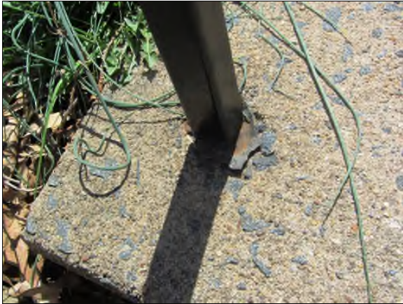
Photo #61. Defective railing socket impounds water causing accelerated deterioration of the metal railing.
