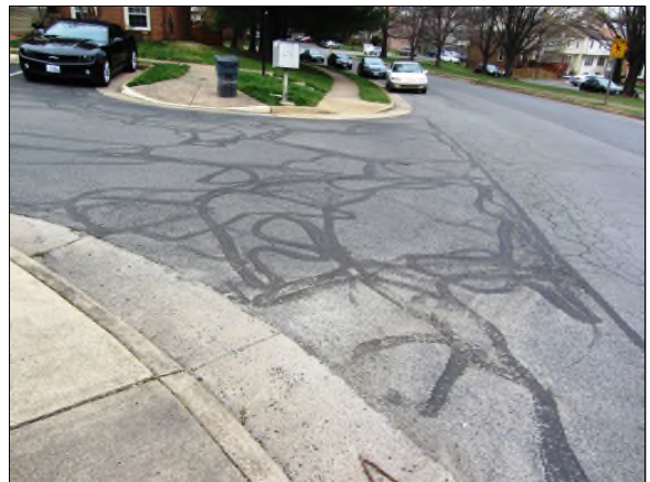
Photo #4. Asphalt pavement at the Grovemore west section.
