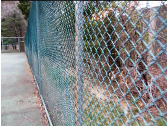
Photo #13. Tennis court fence.
