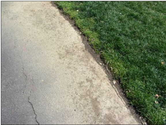
Photo #63. Defective grading adjacent to asphalt trail.
