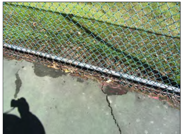
Photo #76. Defective grading at tennis court damages the base materials and bearing soils and causes accelerated deterioration.
