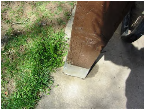
Photo #81. Shed supports in direct contact with the concrete will result in the posts and the structure as a whole, having a limited economic life.
