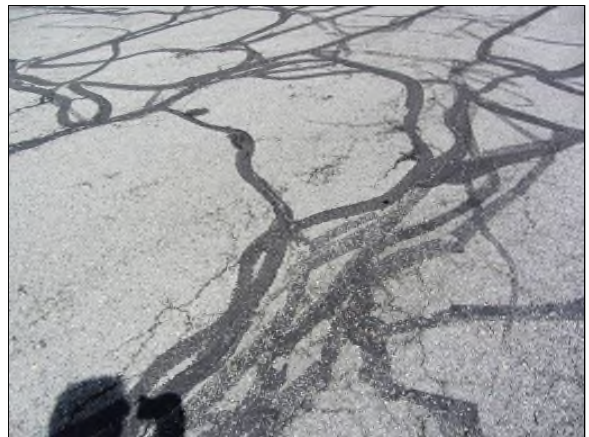
Photo #84. Typical alligatored asphalt pavement with ineffective crack sealing.
