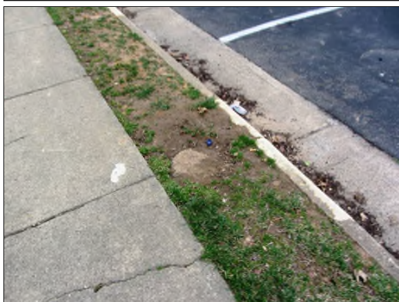
Photo #5. Defective grading and utility access point at incorrect height, Grovemore west section.
