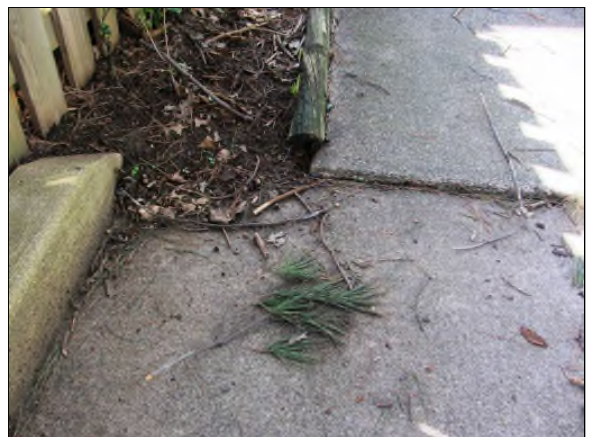
Photo #72. Typical displaced concrete pavement.
