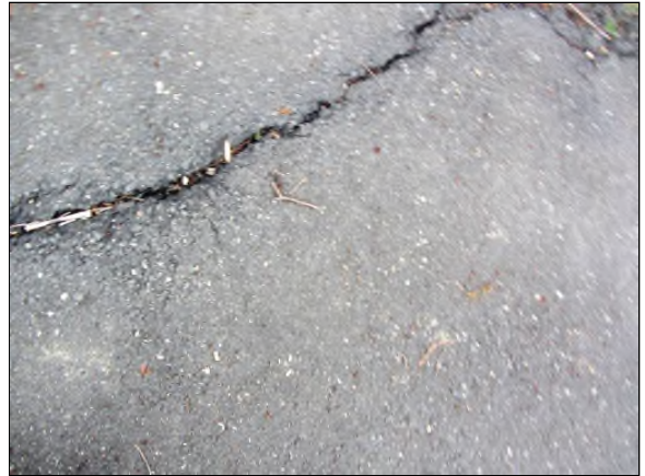
Photo #44. Open crack in asphalt trail.
