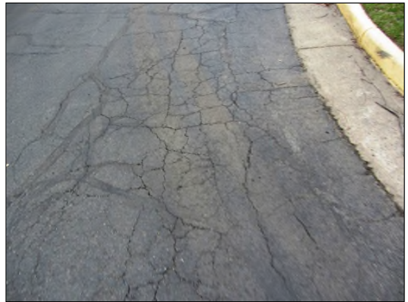
Photo #46. Typical severely alligatored asphalt pavement.
