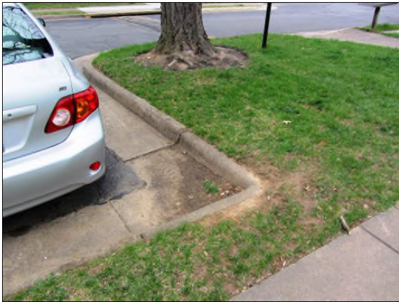
Photo #9. Depressed section of curb & gutter impounds water.
