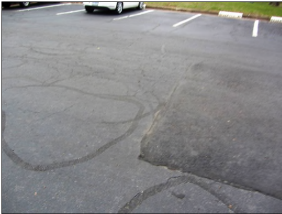
Photo #45. Typical alligatored asphalt pavement and large patches.
