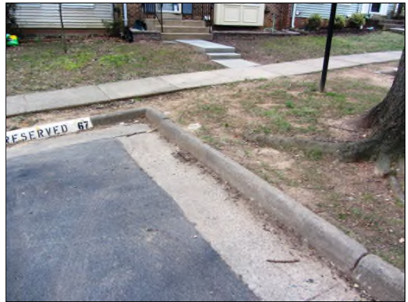
Photo #34. Typical common area without proper ground cover.
