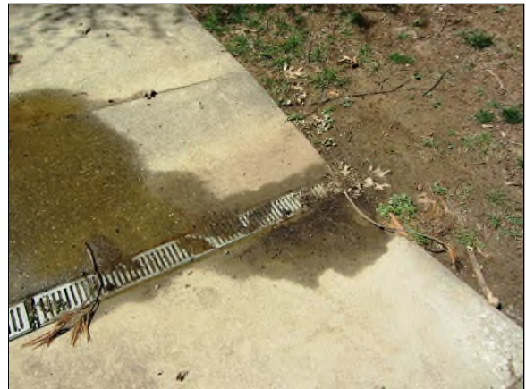
Photo #74. Defective grading (and apparent drainage project) adjacent to concrete pavement.
