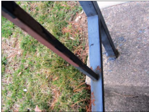
Photo #51. Failed paint system on the metal handrails.
