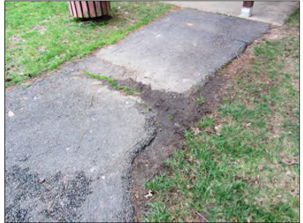
Photo #14. Defective grading adjacent to asphalt trail.
