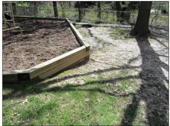
Photo #82. Tot lot border functions as a retaining. Note the lack of a safety railing and ground cover.
