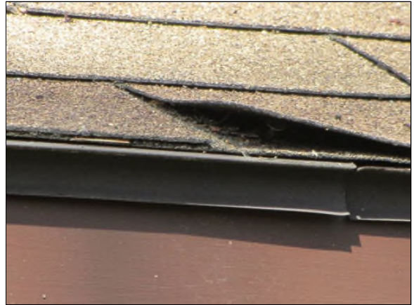
Photo #80. Lifted shingles are prone to wind damage.
