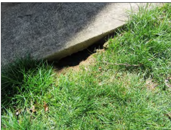
Photo #71. Defective grading directs water under the concrete pavement where it will cause accelerated deterioration.
