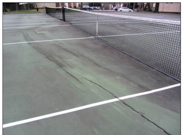
Photo #12. Tennis court with large open cracks.
