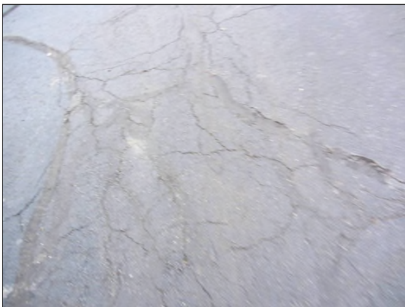
Photo #47. Typical alligatored asphalt pavement.
