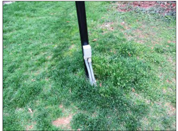
Photo #28. Wiring at streetlight does not date to original construction.
