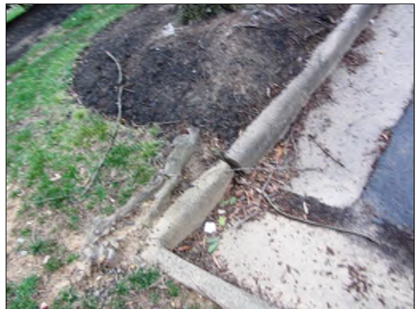
Photo #48. Typical displaced concrete curb & gutter.
