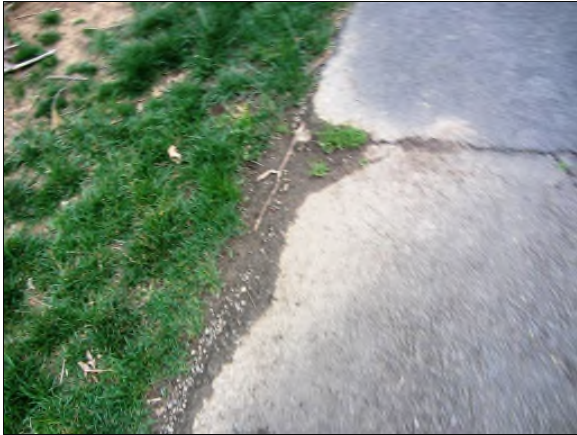
Photo #25. Defective grading adjacent to asphalt trail.
