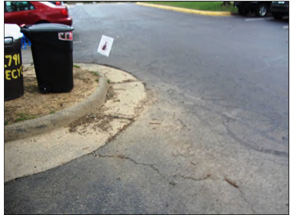
Photo #32. Depressed asphalt pavement and concrete curb & gutter impounds water and likely indicates damage to base materials and bearing soils below.
