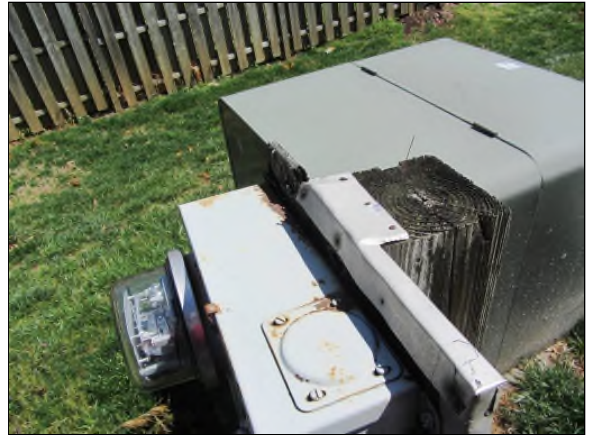
Photo #68. Typical common electrical service.
