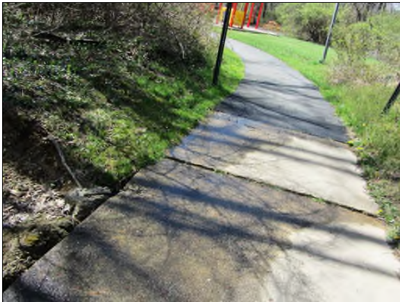
Photo #57. Displaced concrete pavement on the west side of bridge and defective grading adjacent to the pavement create a potential trip hazard.
