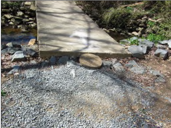
Photo #55. Erosion at east side of bridge.
