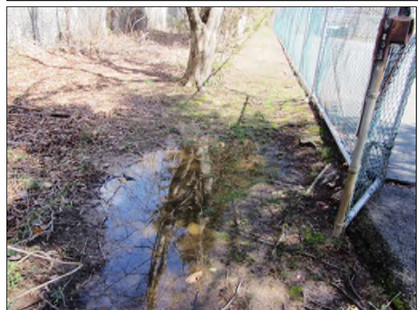
Photo #78. Defective grading at tennis court damages the base materials and bearing soils and causes accelerated deterioration.
