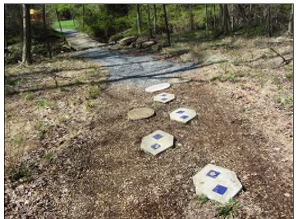
Photo #54. Unsafe walkway leads to the east side of bridge.
