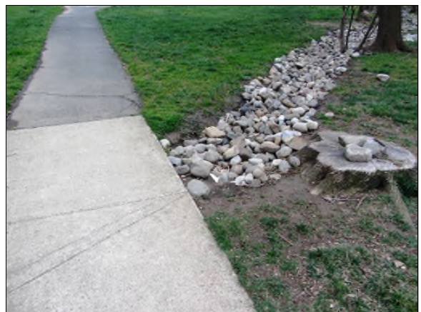
Photo #36. Rock lined drainage swale near the east tot lot.
