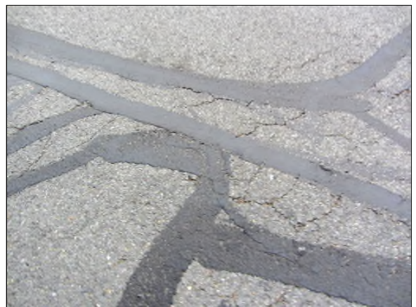
Photo #30. Typical cracked and alligatored asphalt pavement with ineffective crack sealing.
