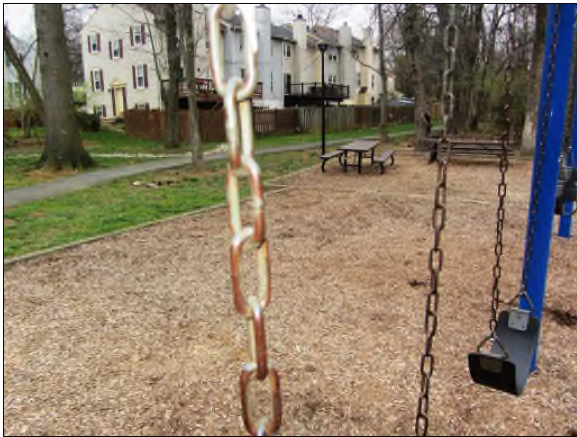
Photo #39. Deteriorated chain, swing in east tot lot.
