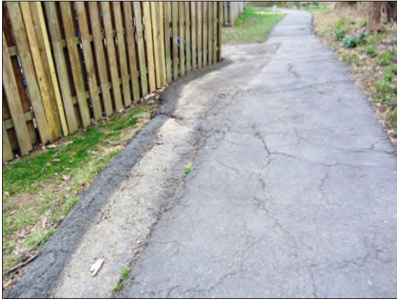
Photo #43. Typical deteriorated asphalt trail.
