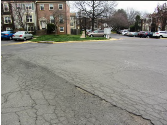
Photo #31. Typical cracked and alligatored asphalt pavement with ineffective crack sealing.
