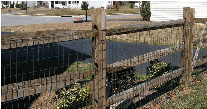
Split Rail Fence with Mesh (from inside)
