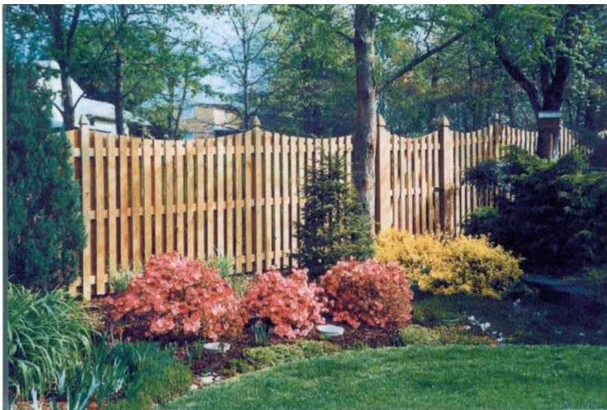
Mt. Vernon Dip Style privacy fence and stockade post (6-ft) – note Offset (overlapping) boards, slat spacing, and design
