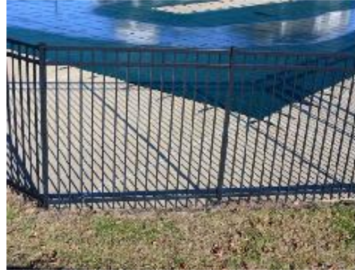
Wrought Iron Fence (see community pool)
