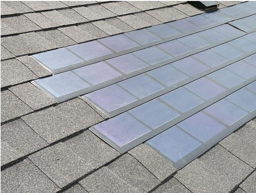
BIPV Shingles example (Uni-Solar; Not sponsored by SMHOA)
