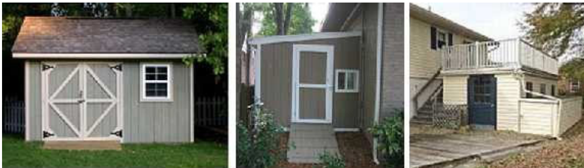
Figure 8: Storage Sheds: Freestanding, Attached to Home, and Under Deck
